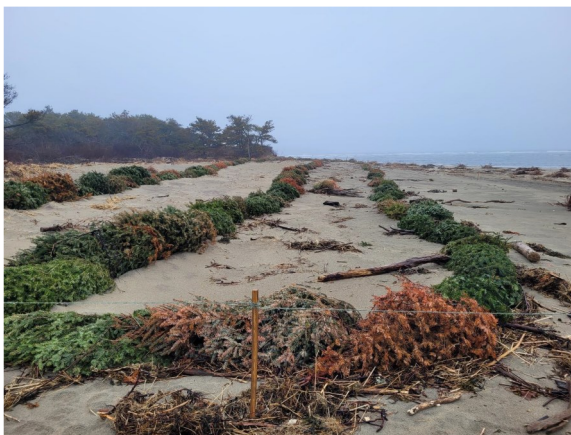
Photo 4: Looking east at center beach at trees about a month after placement. Higher tides are washing sediment into the trees. P. Slovinsky, MGS.
