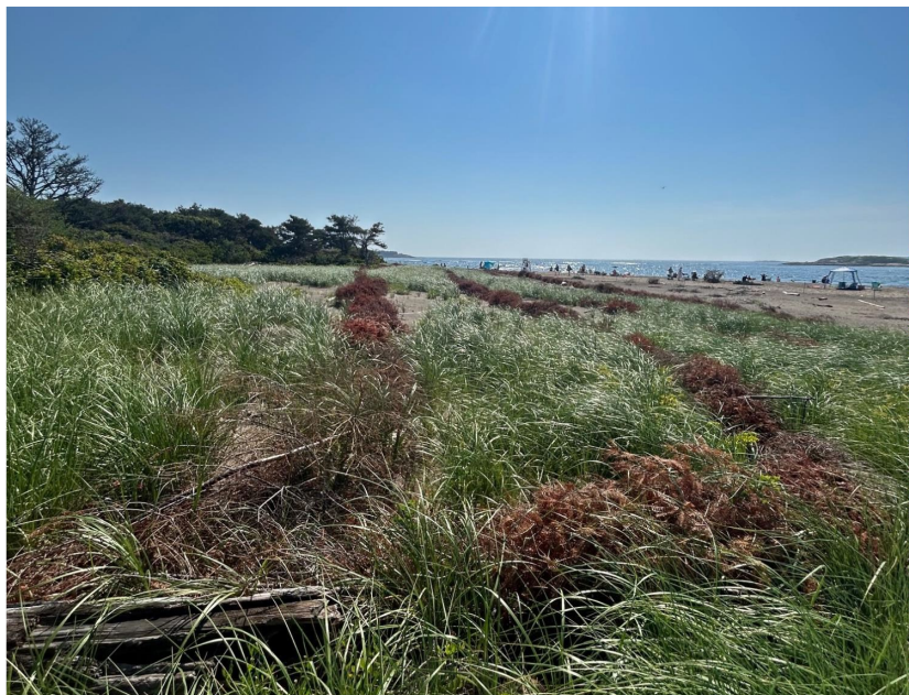
Photo 1 (July 17, 2024 ) Looking east at center beach at trees fourth months after placement. A fourth row was added and is almost completely covered. Note dune grass growth. N. Whiteman, MGS
